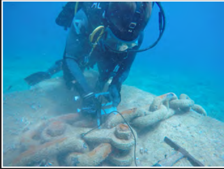
Steelworker Second Class Billy Peacey attached to Underwater Construction Team ONE (UCT ONE) measures the chain on a fleet mooring system sinker in Souda Bay, Crete. Photo by HMC Peter David.
