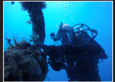
Builder First Class Adam Perry attached to Underwater Construction Team ONE (UCT ONE) takes a caliper measurement on a ground ring beneath a fleet mooring system riser buoy in Souda Bay, Crete. Photo by SWC Liam O’Brien.
