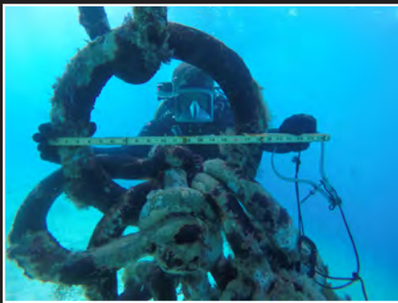
Builder First Class Christopher Kelly attached to Underwater Construction Team ONE (UCT ONE) measures the diameter of a ground ring beneath a fleet mooring system riser buoy in Souda Bay, Crete. Photo by CAPT Brant Pickrell.
