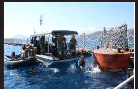
Seabee Divers from Underwater Construction Team ONE (UCT ONE) enter the water to inspect a fleet mooring system riser buoy in Souda Bay, Crete. Equipment Operator Chief Jason Toth front steps into the water while his dive buddy, Builder First Class Carlos Hernandez, looks on waiting to perform their in water checks. Photo by BU1 Christopher Kelly
