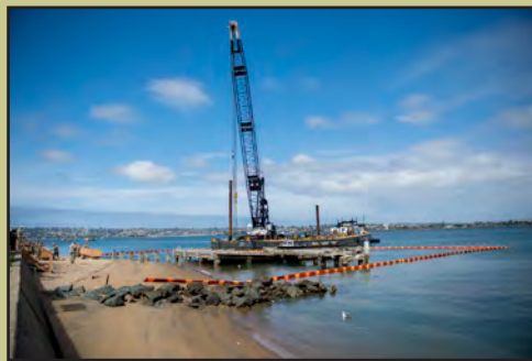
Seabees assigned to NMCB 3 and UCT 2 reconstruct a historic seaplane ramp at Naval Air Station North Island. (Photo by Mass Communication Specialist 2nd Class Carlos M. Vazquez II)
