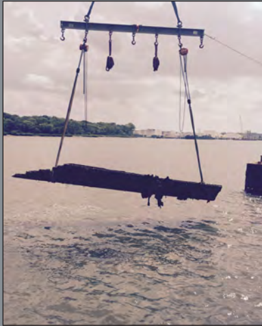
A segmented section of the East Casemate is rigged for recovery.
