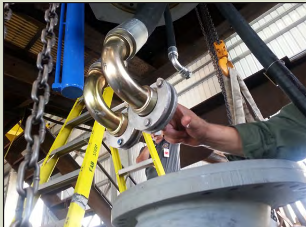
RAT is rigged FWD and AFT with slings. 5 ton chain hoists are connected above to the RAT frame stiffeners. RAT stem to lower unit is disconnected and lowered for removal. As soon as RAT motor is on surface, divers will install a cofferdam over the hydraulic hoses and bolted to stem flange and then dewatered. Reinstallation is completed in the reverse.
